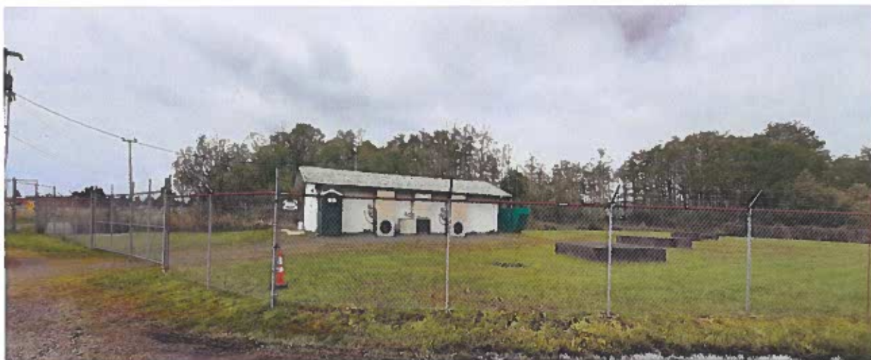
Communications Hub Building
