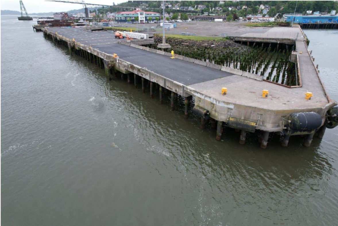
Overall view of Pier 1, looking east.
