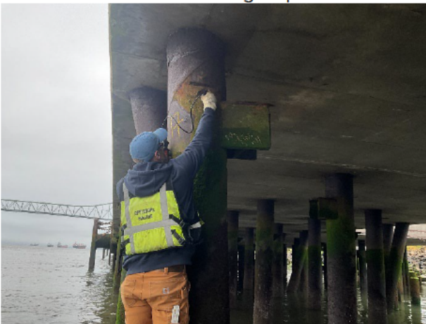
Photo 5: Engineer taking thickness reading at Pile 17:A.
