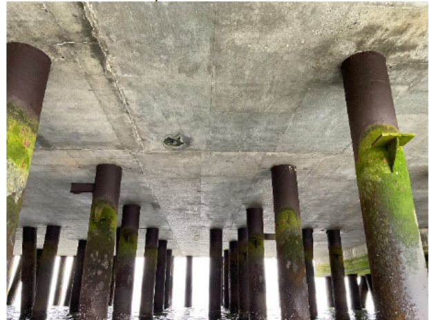
Photo 4: Typical underdeck at Bent 34.
