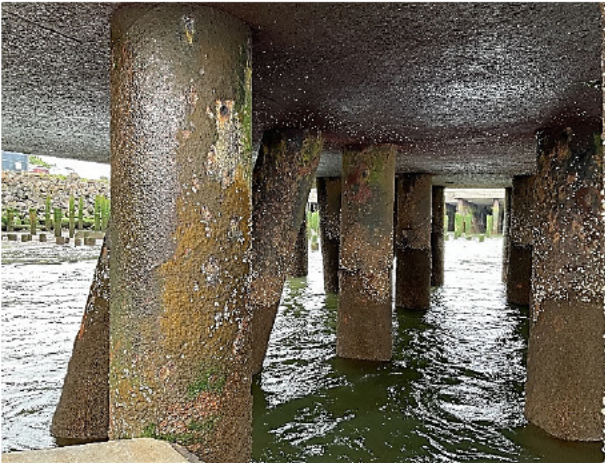
Photo 3: Piles at the breasting dolphin.
