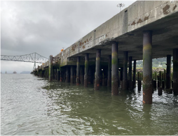
Photo 1: Looking east from Bent 7.
