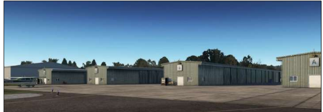
T-Hangar Rows at the Airport
