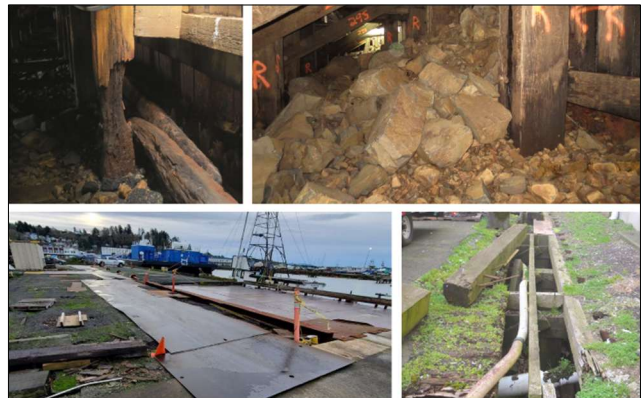
Pier 2 West Dock & Pier Conditions
