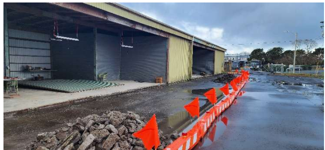
T-Hangar Row A Rehabilitation was completed in FY2025-26
