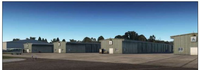
T-Hangar Rows at the Airport
