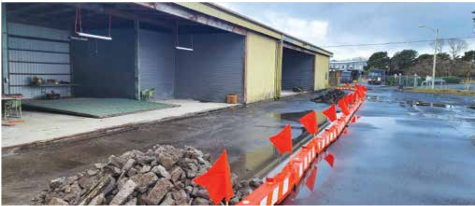
T Hangar A Row—Before and during rehabilitation project.
