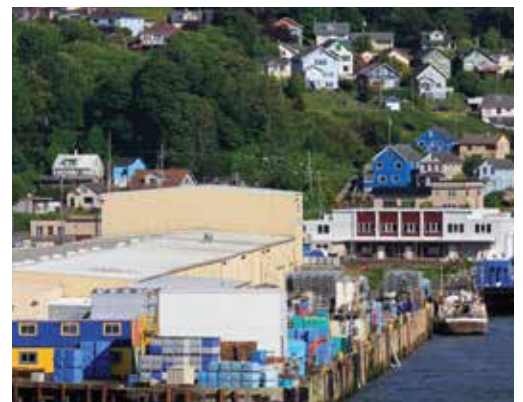
Above: Pier 2 West
