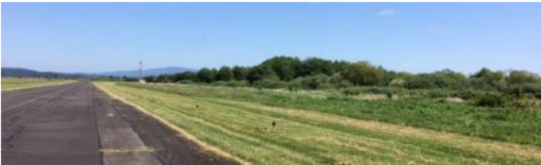
Tree and shrub penetration of the Transition Surface on SE side of RWY 26
