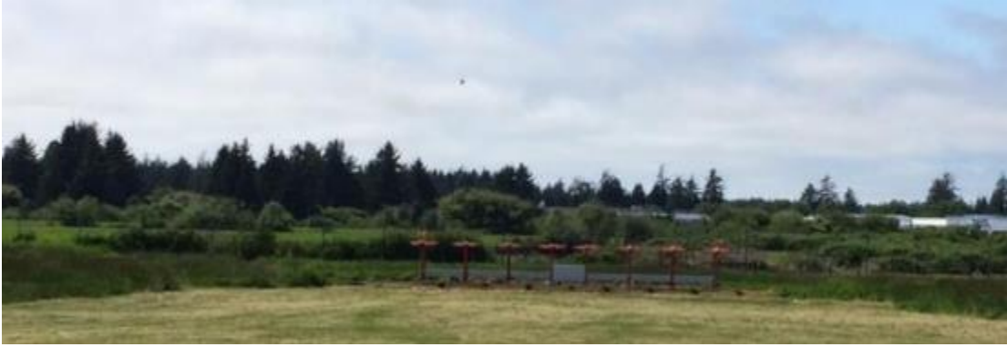
Tree and shrub penetration of the Approach Surface on the west side of RWY 8.
