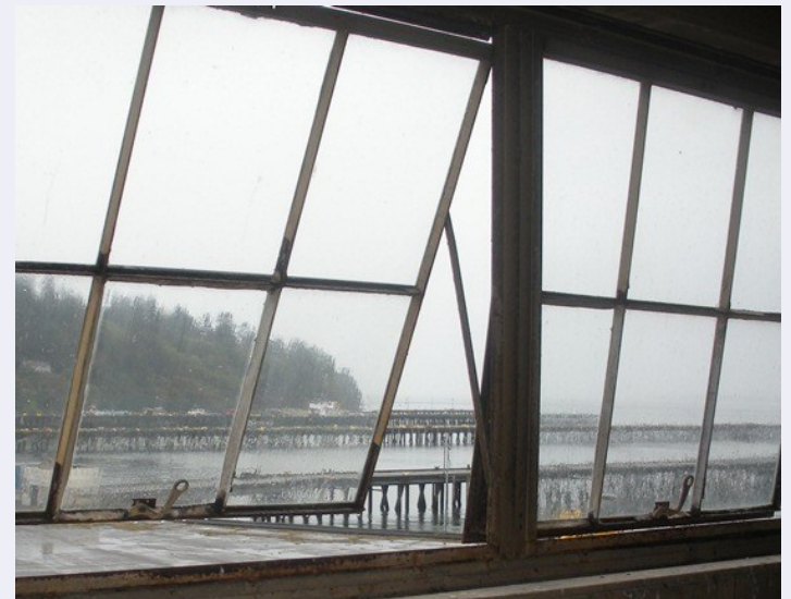
3 Hangar way | Office space windows and views
