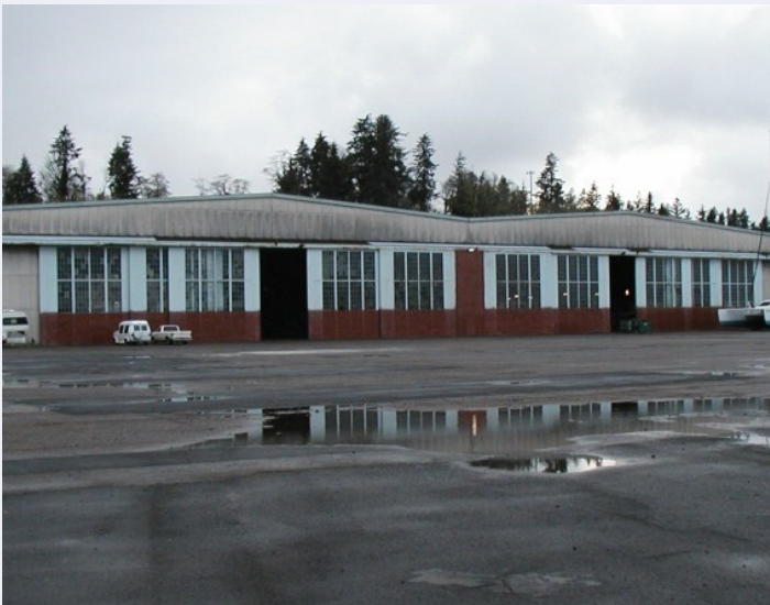
3 Hangar Way | Hangar 3 and tarmac space
