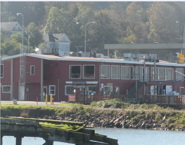
300 Industry Ave | North side of building
