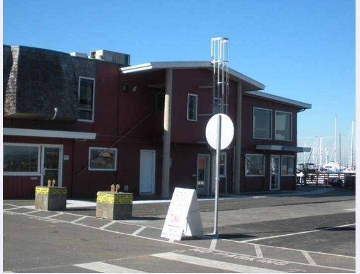
300 Industry | East side of the building
