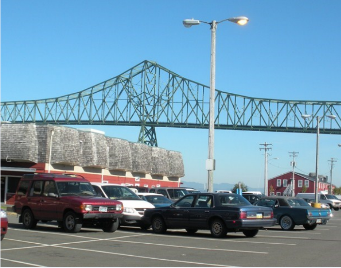
300 Industry Ave | South side of building
