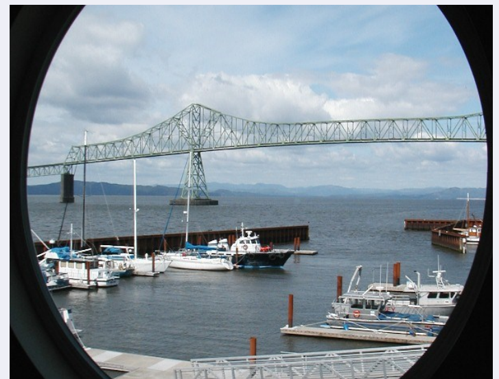
10 Pier 1 | View from stairwell porthole
