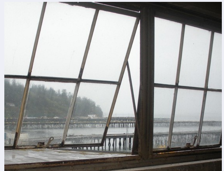
3 Hangar way | Office space windows and views
