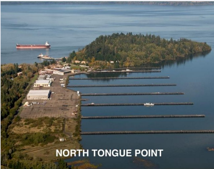
3 Hangar way | Six 1500' long piers and access to the nearby shipping channel
