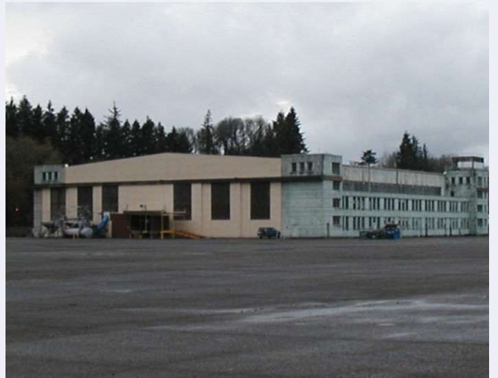
3 Hangar Way | Hangar 2 and tarmac
