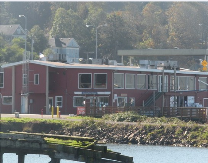
346 Industry Ave | North side of building
