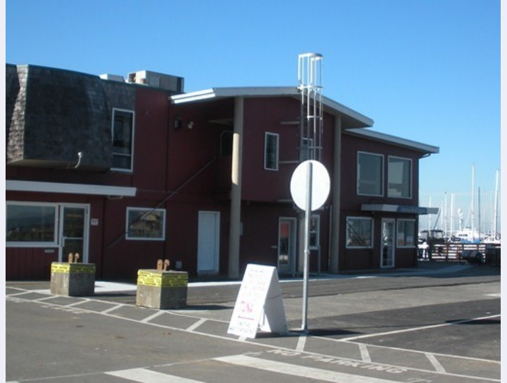
346 Industry | East side of the building
