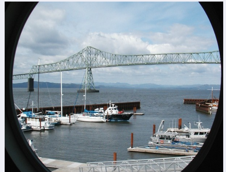
10 Pier 1 | View from stairwell porthole
