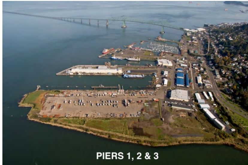
Figure 7 – Port of Astoria Piers 1, 2 & 3 and Uplands
