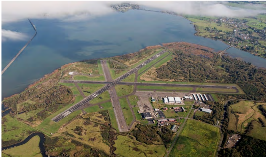
Figure 5 – Aerial View of Astoria-Warrenton Regional Airport
